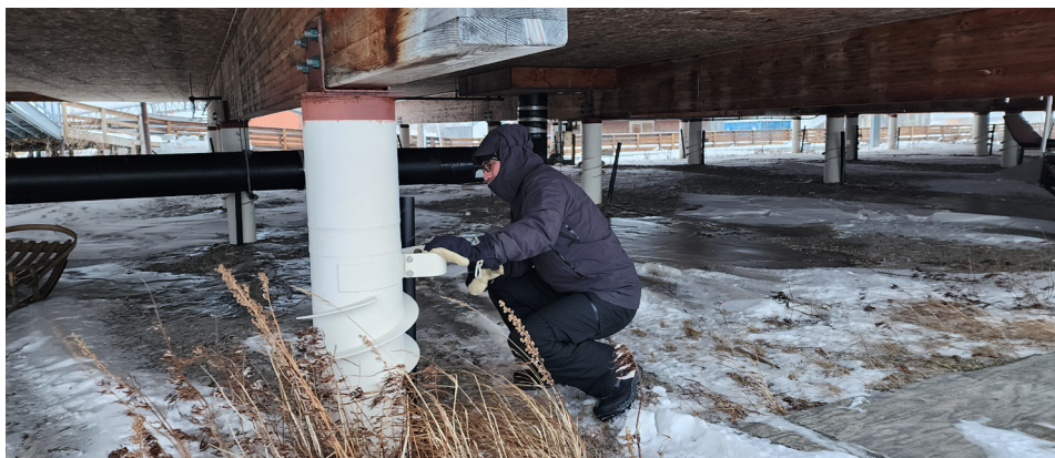
Tyler Goldade, Facility Condition Assessment program manager at Tribal Development Partners, examines foundation and structural components beneath a tribal facility during an assessment. Facility Condition Assessments help Tribal organizations document long-term capital needs and support infrastructure planning under Section 105(l)
